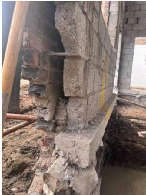
Original house wall construction showing cavity wall present 12 May 2016
