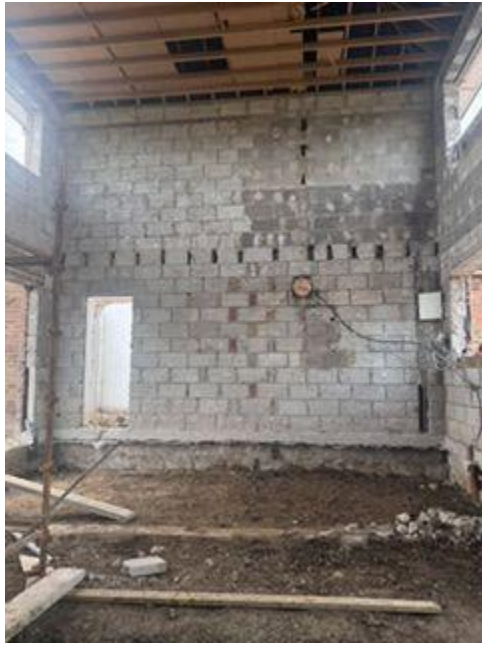
Original house - stripped for refurbishment 12 May 2016
