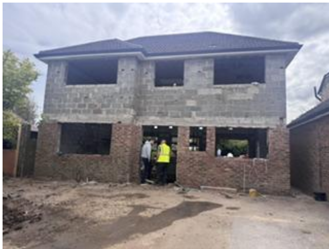
Original house - stripped for refurbishment 12 May 2016
